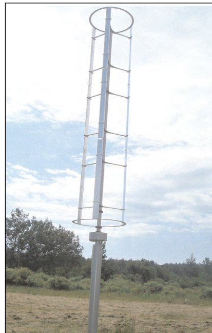
The Mille Lacs Band is among the first in Minnesota to install a new type of vertical wind turbine called the Windspire.
