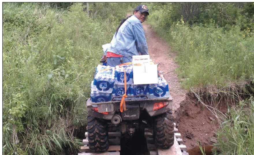
Mille Lacs Band Department of Natural Resources staff built a temporary bridge so that they could deliver water and check on local residents during the flood in June.
